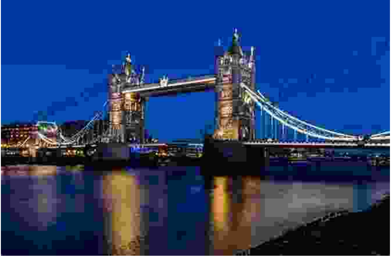
Tower Bridge Detail
